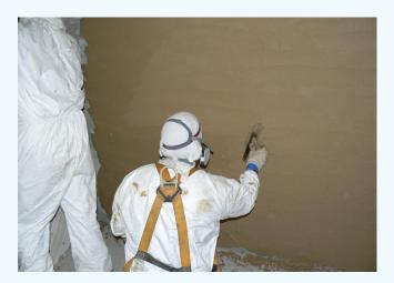
**SewerGard® No. 210S - Sprayable** formulation is fiber-reinforced for a high degree of durability. No. 210S allows quick installation by a single 60-mil coat when applied by standard airless equipment. It is ideal for large-scale applications.
