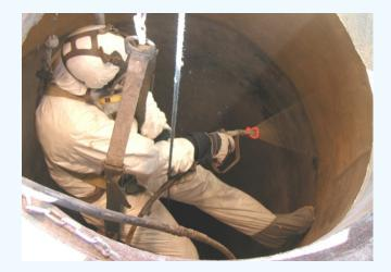
**SewerGard® No. 210RS - Rotary Spray** formulation is a pumpable grade of SewerGard® specifically designed to line the interior of manholes from street level. No. 210RS is applied at 60-125 mils using typical rotary application equipment.
