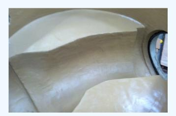
Each formulation of SewerGard® provides an impermeable, high strength, corrosion-resistant lining for structures subject to infiltration and attack from hydrogen sulfide and acid generated by microbiological sources.
