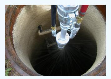
**SewerGard® No. 210X - High-Strength** formulation is a highstrength lining that enables high-build capabilities wherever extreme corrosion conditions exist. It is easily applied by plural-component or conventional airless spray equipment.
