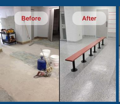
The KEY URECON Chip-100, a urethane-modified cementitious floor system finished with a decorative broadcast flake, provides many advantages to designers and contractors over a standard epoxy chip floor.
